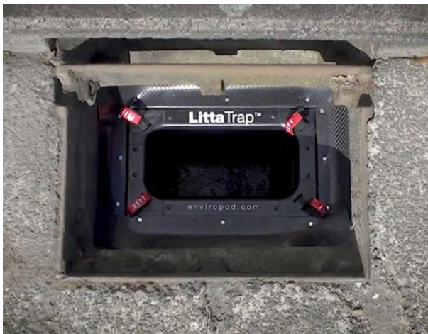
Cleaner waterways: The Council is trialling the use of litter collection basket at stormwater drains.
