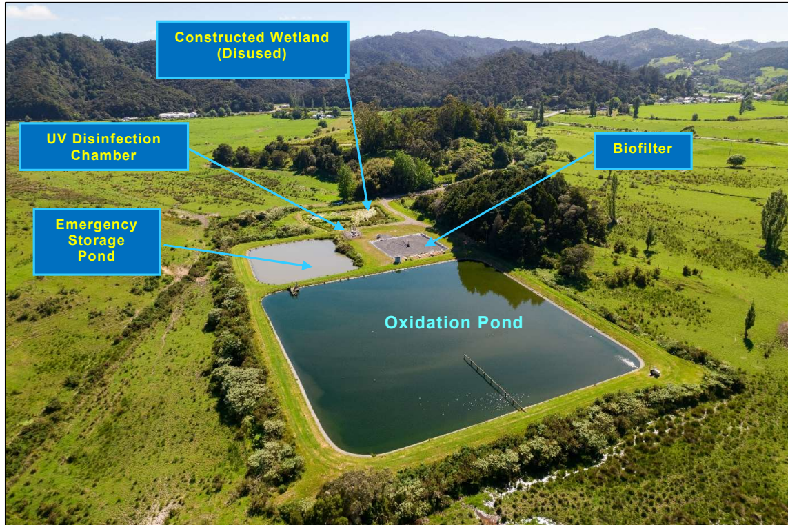
Figure 4: Photo of Kāeo WWTP (Source: Aerial Vision Ltd, 28 November 2021).
