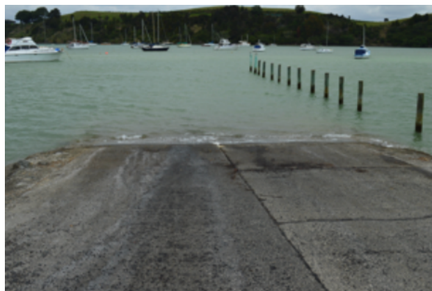
Figure 3 - Ramp and Fender Piles
