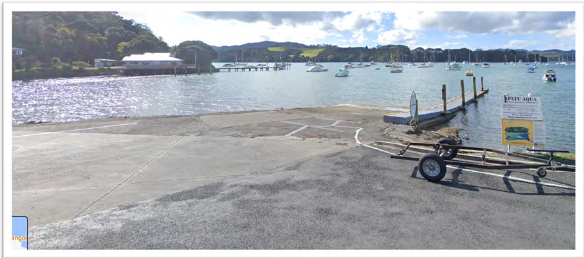
Figure 3 - Ramp and Jetty and Pontoon
