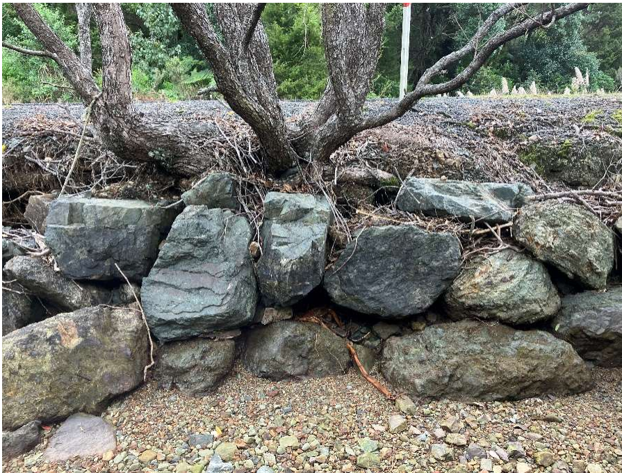
Figure 9. Rock armour adjacent to culvert.
