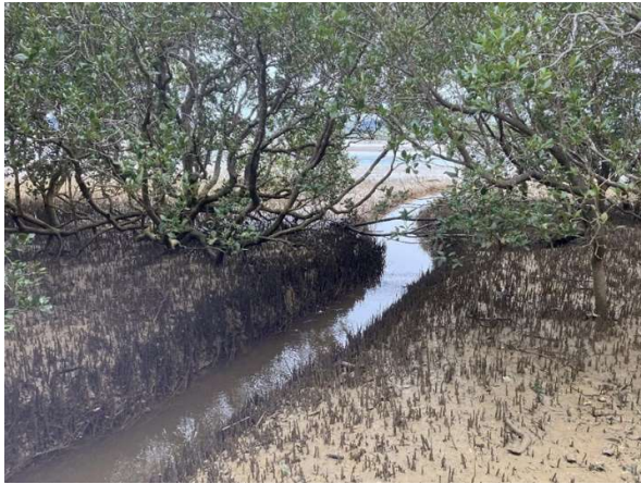
Watercourse 1 downstream of the culvert
