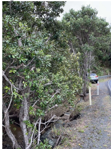
Vegetation adjacent to the south of the culvert
